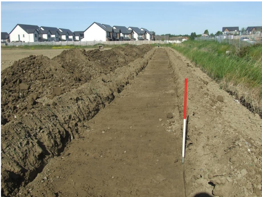
Plate 35: Field 9 Test Trench 8 looking west
