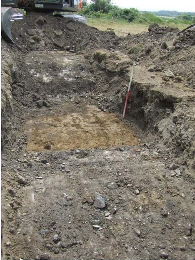
Plate 9: Field 4 mid-excavation of Test Trench 2 looking south
