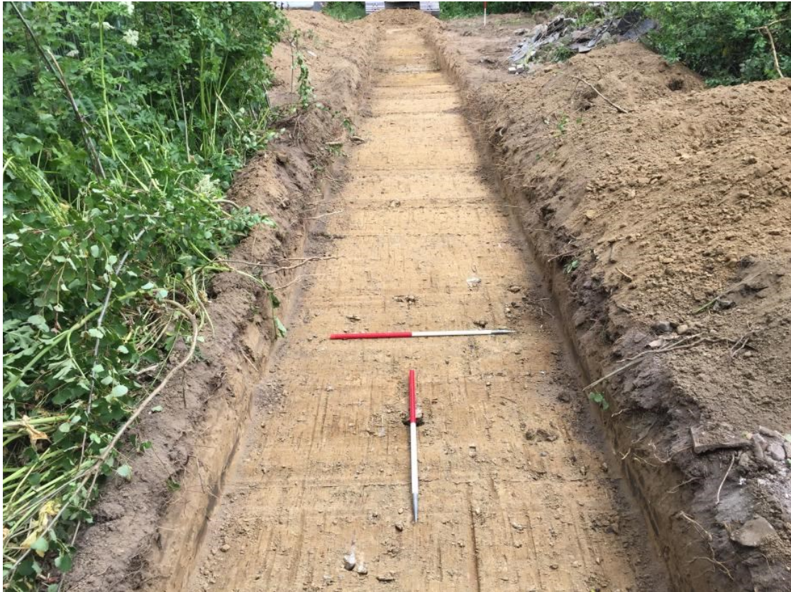
Plate 28: Field 7 Test Trench 1 looking east
