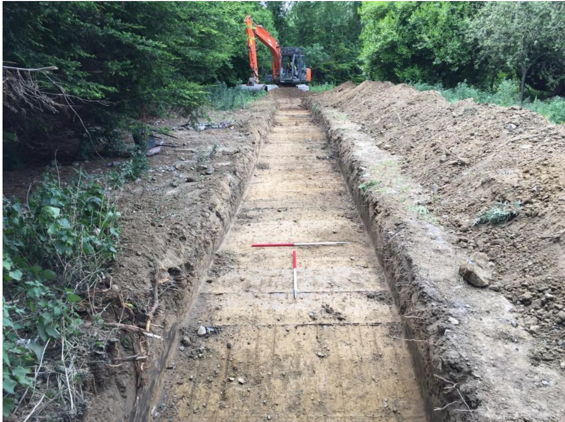
Plate 30: Field 8 Test Trench 1 looking west
